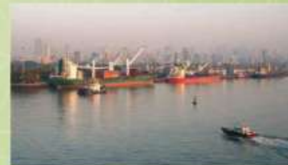
*International Cruise Terminal (ICT) (Ballard Pier)
